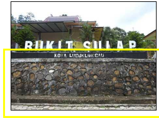
Figure 1. Stone retaining wall of Bukit Sulap
